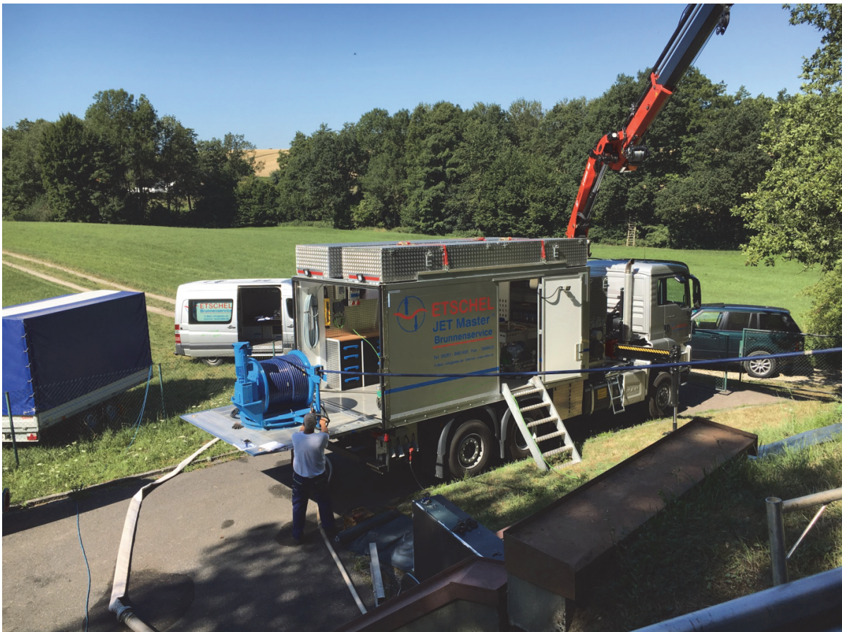
Figure – Mobile unit for water well rehabilitation and water well development
